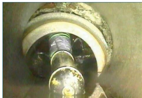
Ground settling over time can cause sewer pipes to become disjointed, causing infiltration, blockages, and reduced pipe capacity.
