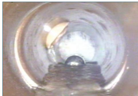
A sewer lateral (the pipe that connects a private home or business to the main sewer line in the street) intrudes into the main sewer line. This intrusion can cause debris to get caught, leading to blockages and backups into homes or onto the street.
