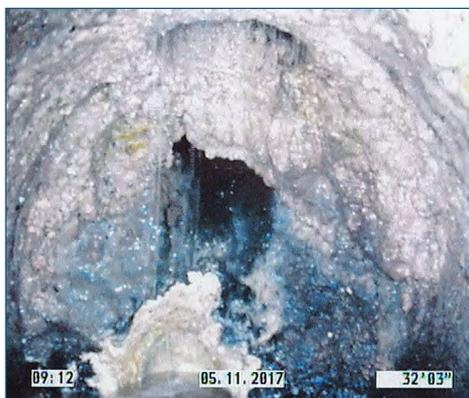
When warm, FOG is typically in liquid form. However, once cooled, FOG hardens and decreases capacity of the sewage pipe. This can lead to backups into homes and onto streets.
