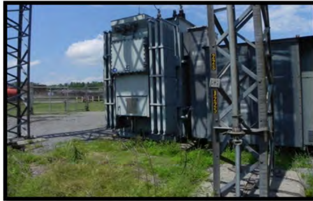
46kV to 4160V Power Transformer
