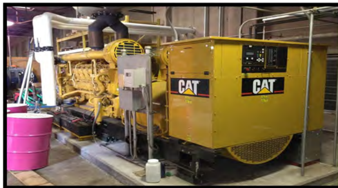
2250kW, 4160V, Standby Diesel Engine Generator
