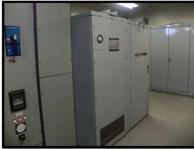
4160V Primary Switch and 4160 to 480Y/277V Unit Substation Transformer
