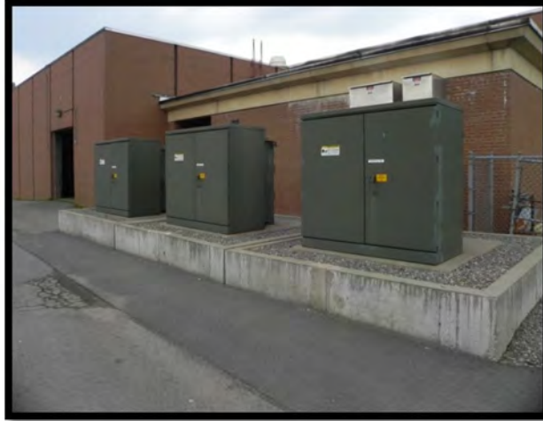
Exterior Pad Mount 4160V to 480V Power Transformers
