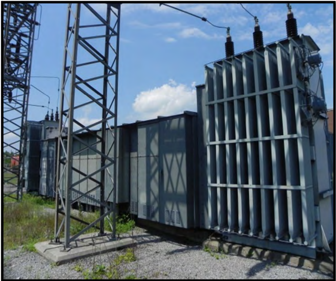
Existing Outdoor Main Unit Substation 46kV to 4160V
