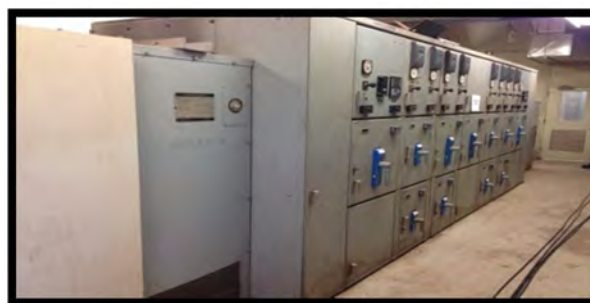
Double-Ended Unit Substation
