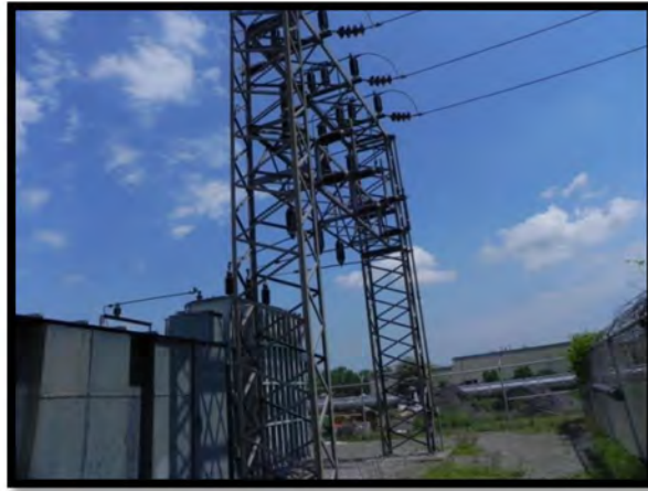
46kV Group Operated Air Break Switches, Vertical Mount Disconnectable Power Fuses and Lightning Arrestor
