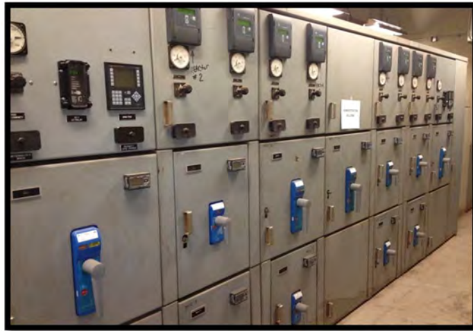
480Y/277V Switchgear Lineup
