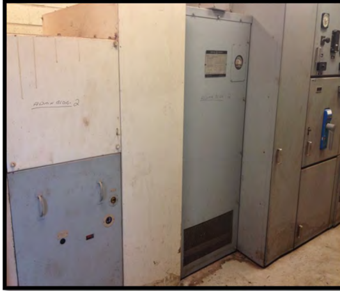
4160V Primary Switch and 4160V to 480Y/277V Power Transformer
