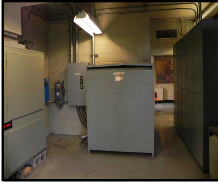
Interior 4160V to 480Y/277V Transformer
