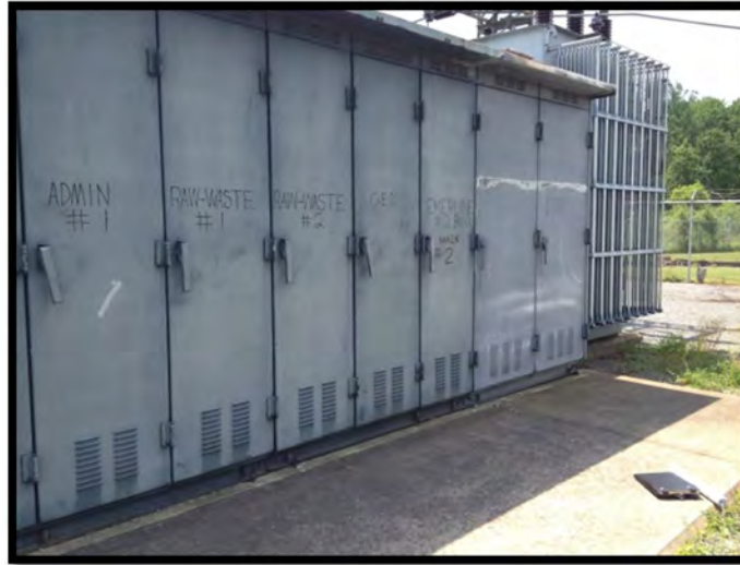
4160Y/2400V Metal-Clad Switchgear Lineup
