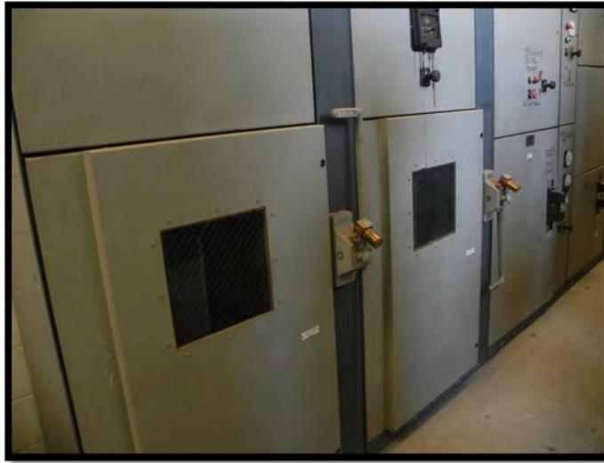
4160V Primary Selector Switches
