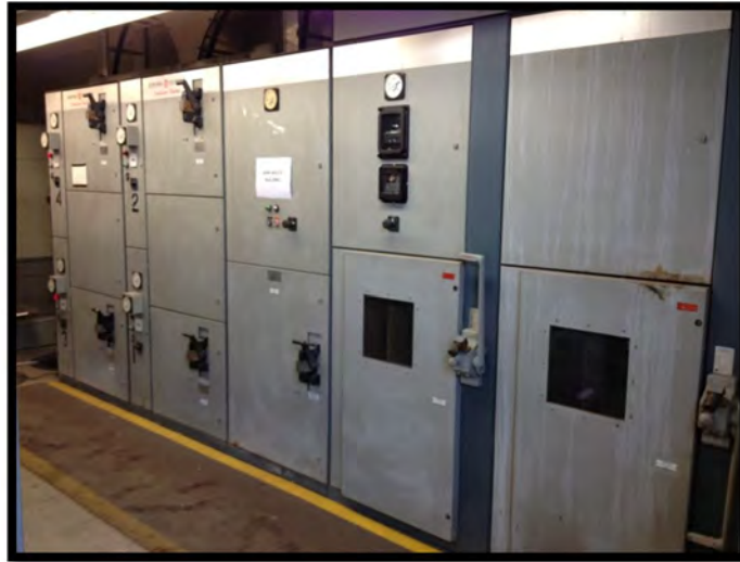
Medium Voltage Motor Control Switchgear
