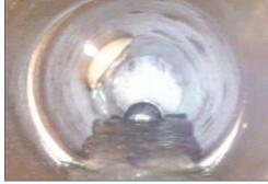
A sewer lateral (the pipe that connects a private home or business to the main sewer line in the street) intrudes into the main sewer line. This intrusion can cause debris to get caught, leading to blockages and backups into homes or onto the street
