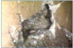
Cracks and holes such as these in sewer pipes enable sewage to leak out and groundwater to infiltrate, leading to overflows during heavy rains and snow melts. This condition eventually leads to a pipe collapse.
