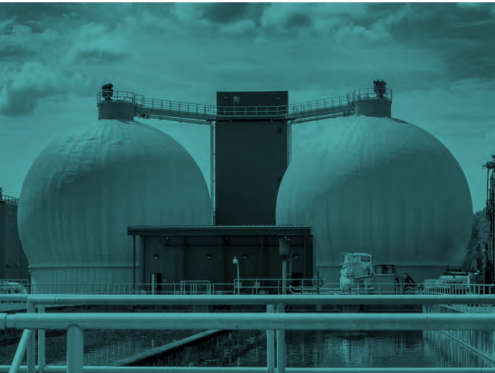
Pictured above is the newly-constructed anaerobic digesters.
