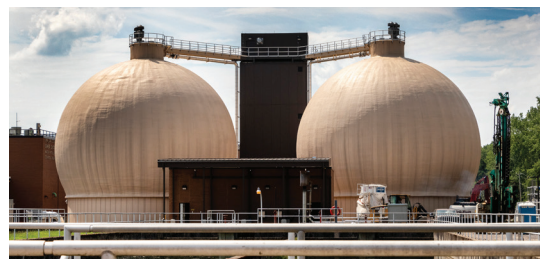
Installation of new aerobic digesters increase capacity of solids and reduce energy costs.
