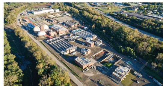
Upgrades at the Oneida County Water Pollution Control Plant (WPCP) include energy recovery capabilities, food waste receiving facilities, a new 27 MGD pump station/screen facility for sanitary flow, and a refurbished 49 MGD pump station for City of Utica Flows.
